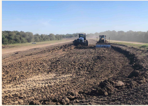
Raising a levee with new fill.
